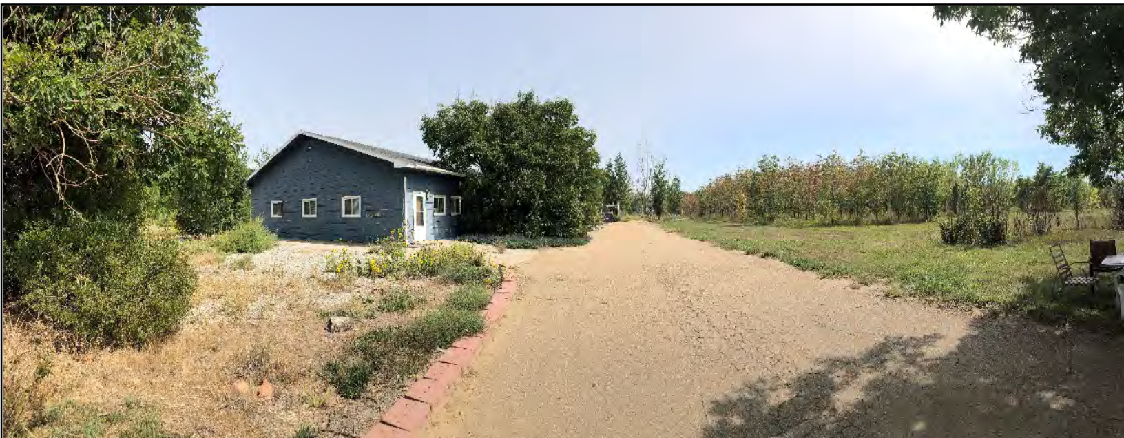
Photo 2. Office building and entry area. (9/14/20).
