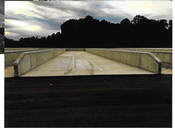
CASP SYSTEM: COVERED AERATED STATIC PILES - Feedstock is covered in a concrete bunker system process, creating a closed system that fully contains leachate and minimizes odors.
